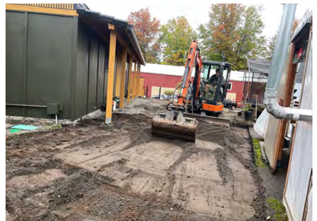
Ty Card donating his time leveling the new addition.
