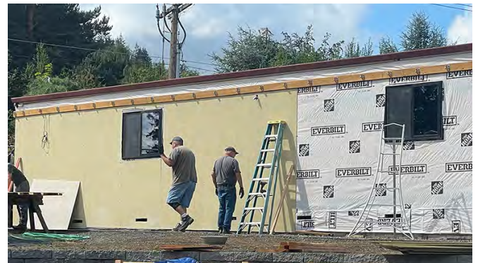
Hardiplank siding going up, a heavy lifting and cumbersome job.
